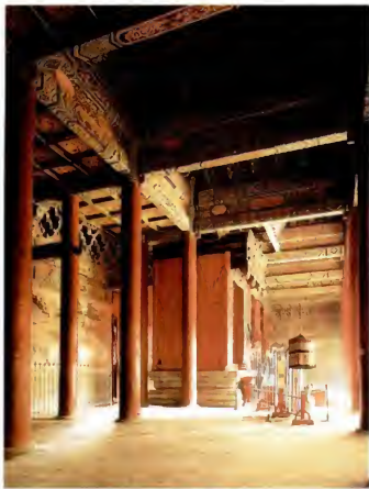
Fig. 12 Dai Miao (Dai Temple), a Qing dynasty structure on Tai Shan (Mount Tai, the Eastern Peak; also called Dongyue), Shandong province.
